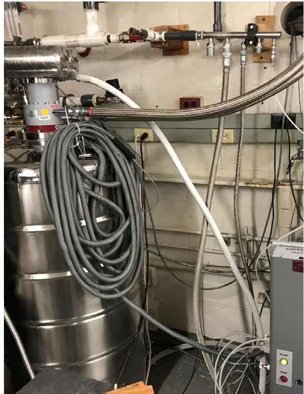
Fig 4 Image of the LHEP while transferring. You can see that the frost on the recovery line carrying return gas from the transfer line extends quite far
